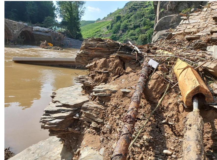
Destroyed Infrastructure in Ahrtal/Germany
